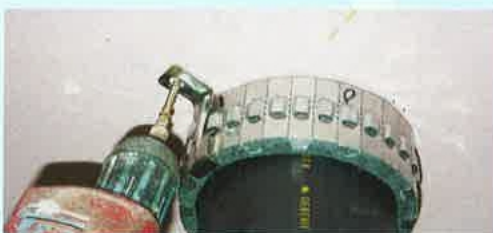
Secure remaining brackets to wall/floor.
