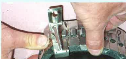
Fit onto the pipe and use first bracket to joint ends.
