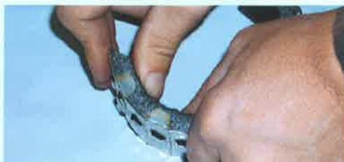
Shape the required collar to suit the pipe.
